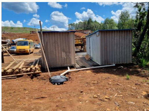
Biodigestor instalado
